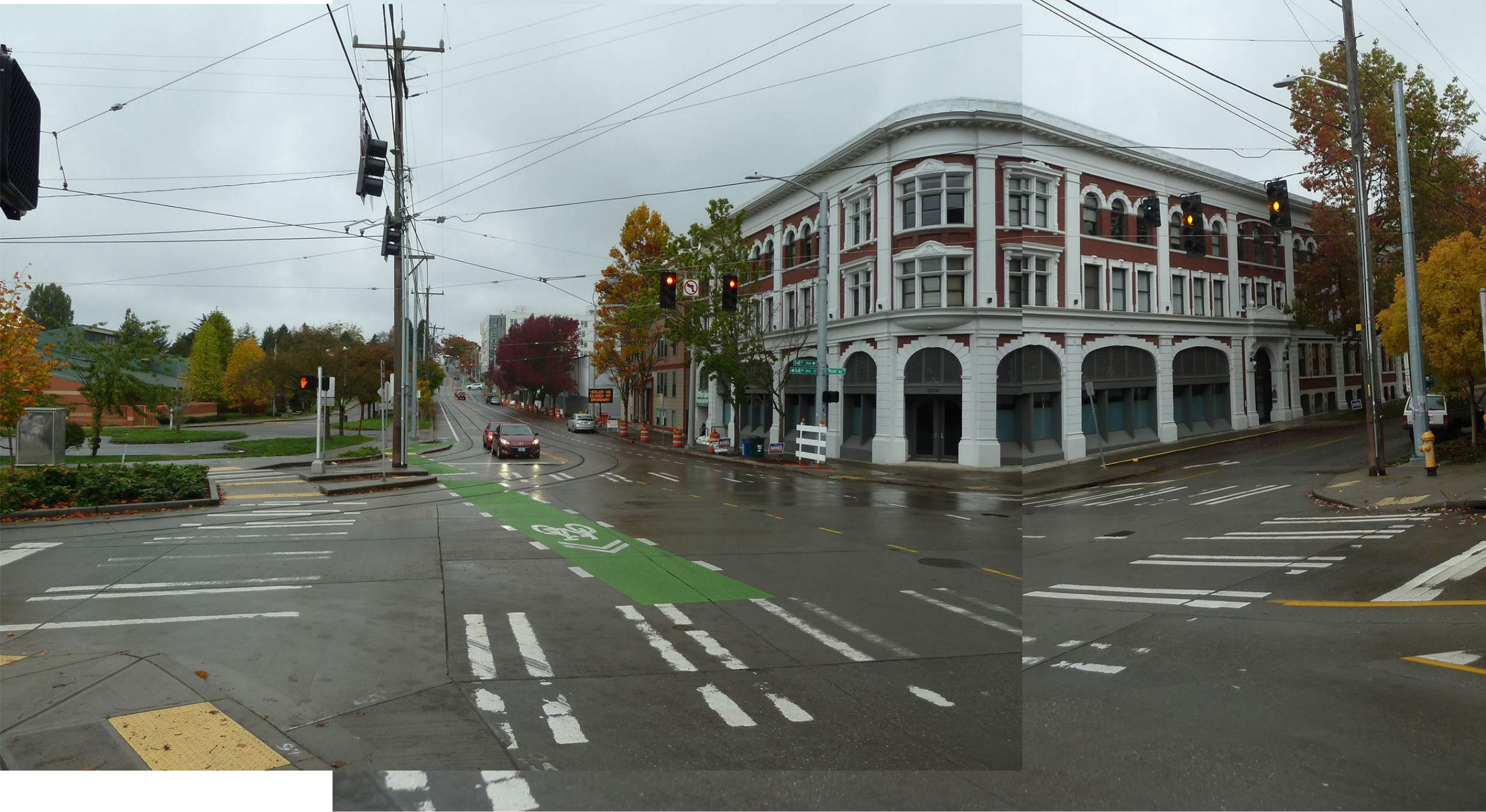
east of site - looking west
